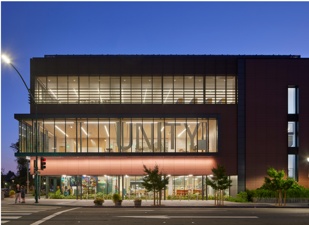
Activating a Downtown Streetscape
