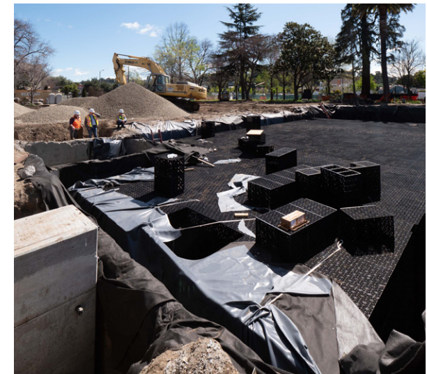
Cistern Being Installed
