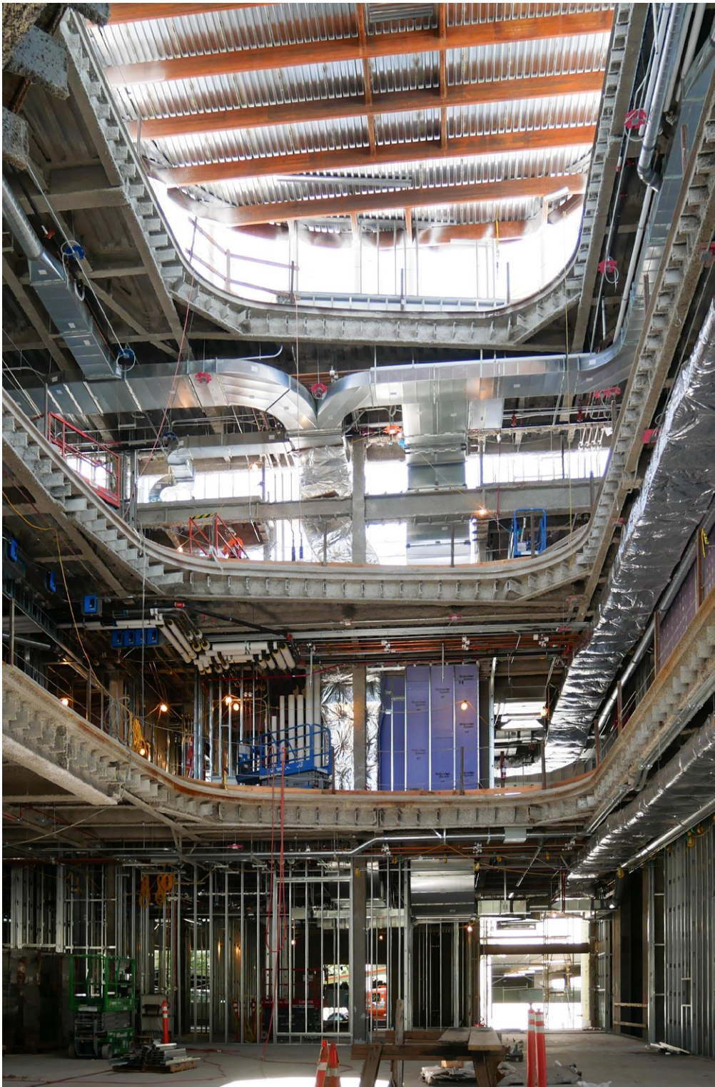
Efficient Dedicated Ventilation & Clerestory Daylighting
