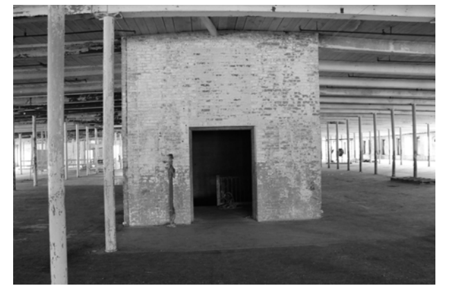
The seven foot east-west grid of columns are used and edited in a variety of ways to define space while permitting passage.
