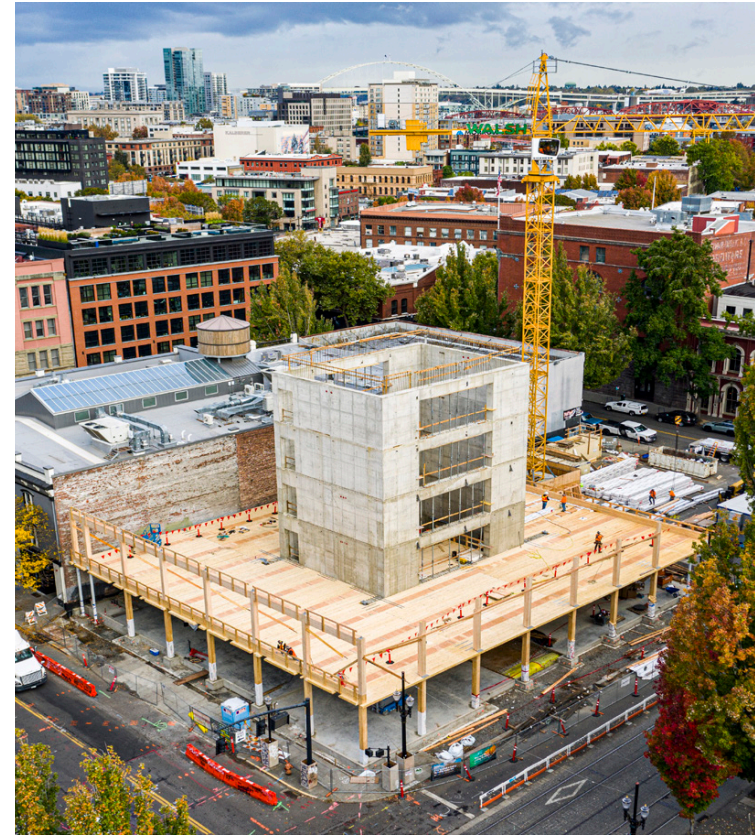
A densely reinforced shear-wall core surrounded by glulam columns and beams and concrete-topped CLT floor diaphragms allow the building to survive a major seismic event.
