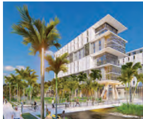
New Construction WSHP | Central Plant
