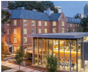
Renovation + Addition 4-Pipe Fan Coil | Central Plant
