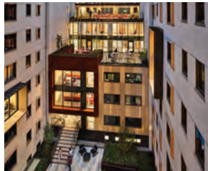
Renovation + Addition WSHP | Existing Boiler Reuse
