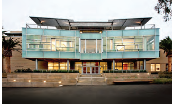
David Allan Hubbard Library Renovation + Addition Fuller Theological Seminary | Pasadena, CA 2009 | WM+P with House + Robertson Project Manager / Project Architect
