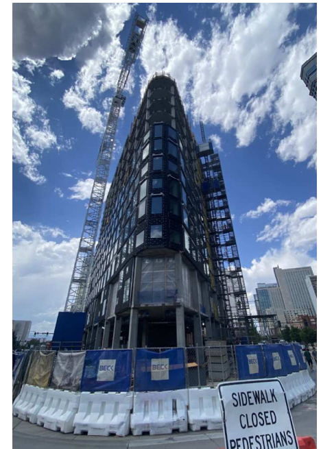
Exterior wall before cladding
