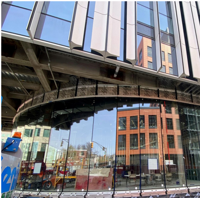
Innovative glass wall spanning 25 feet w/o mullions.
