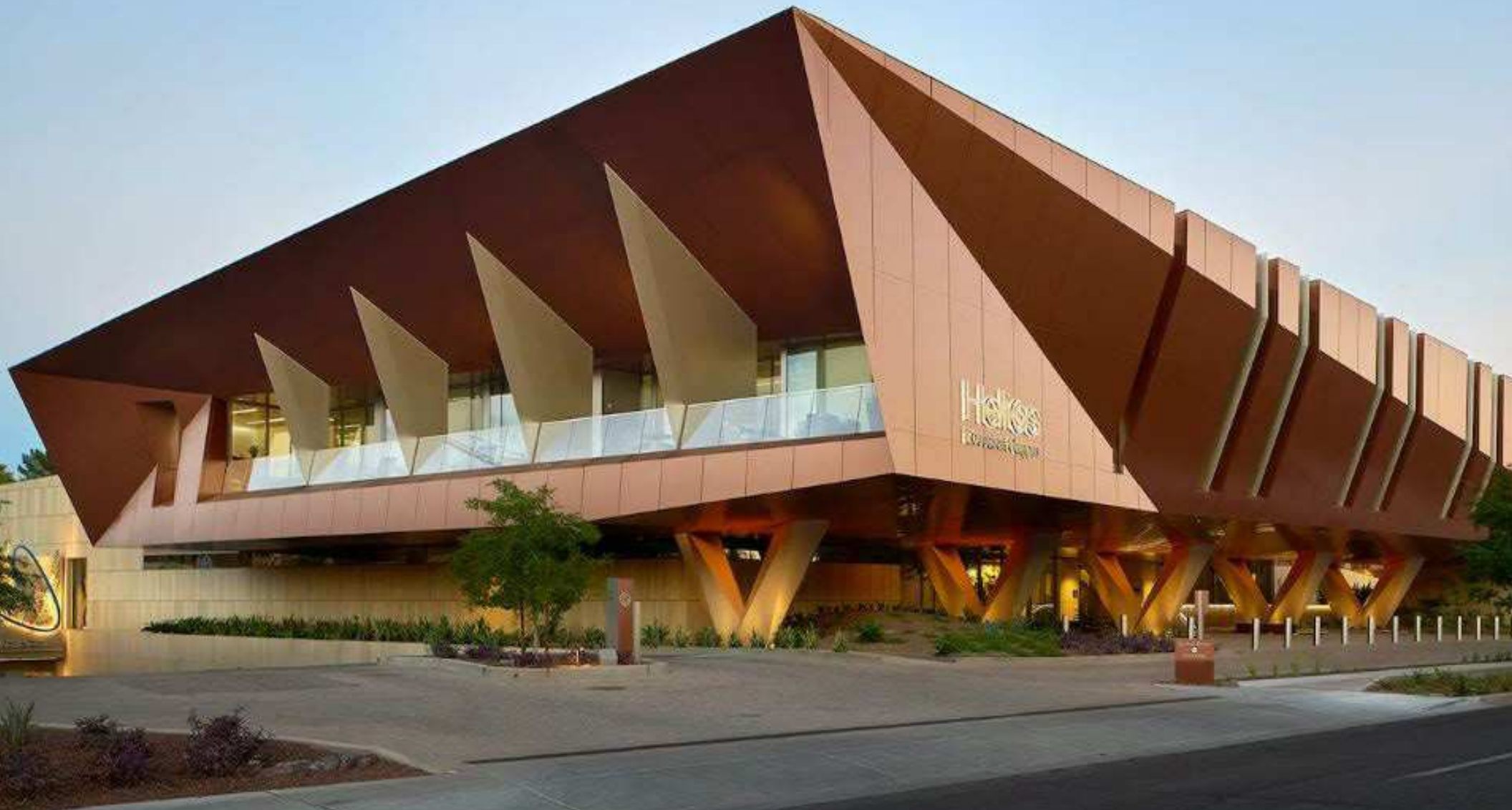
Helios Education Foundation Net-Zero headquarters self-shaded facade - Phoenix, AZ
