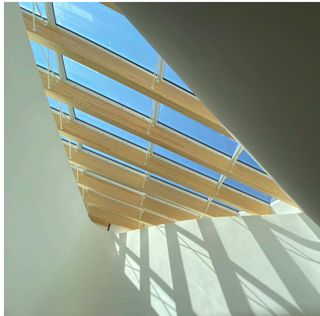
Timber skylight at central atrium
