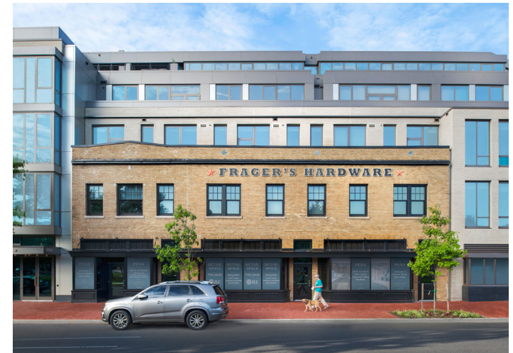
The team preserved and restored the original facades of historic Frager's Hardware while transforming the site into a 34-unit mixed income residential building.
