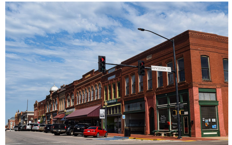
100 Block West Oklahoma Avenue, North Side: All 12 buildings had metal slipcovers when Frantz provided design assistance.
