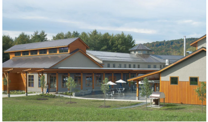
King Arthur Baking Company in Norwich, Vermont, designed by Diantha Korzun while working at TruexCullins. Photo Credit: Jim Westphalen.
