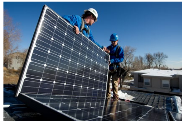
Rigid solar PV panels being installed on a roof.
