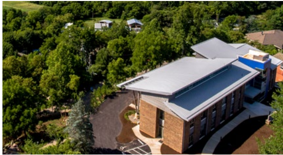
Solar-ready architecture featuring a long east-west axis with adequate south-facing roof for solar PV
