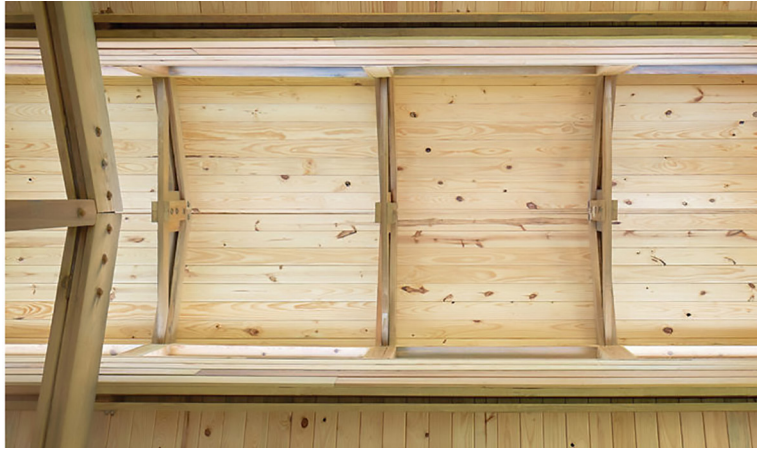
Figure 6: Use of mechanical fasteners and minimal use of adhesives make it easier to adapt the building later because assemblies can be taken apart without damage and even, in some cases, be reassembled in another part of the building. Dixon Water Foundation Josey Pavilion. Photo Credit: Casey Dunn
