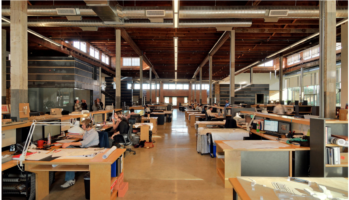
Figure 2: 2015 COTE Top Ten Recipient Hugh Warehouse by Overland Partners showcases clear spans, regularly spaced structural elements, and mechanical fasteners. Image: Dror Baldinger, AIA and Scott Adams, AIA
