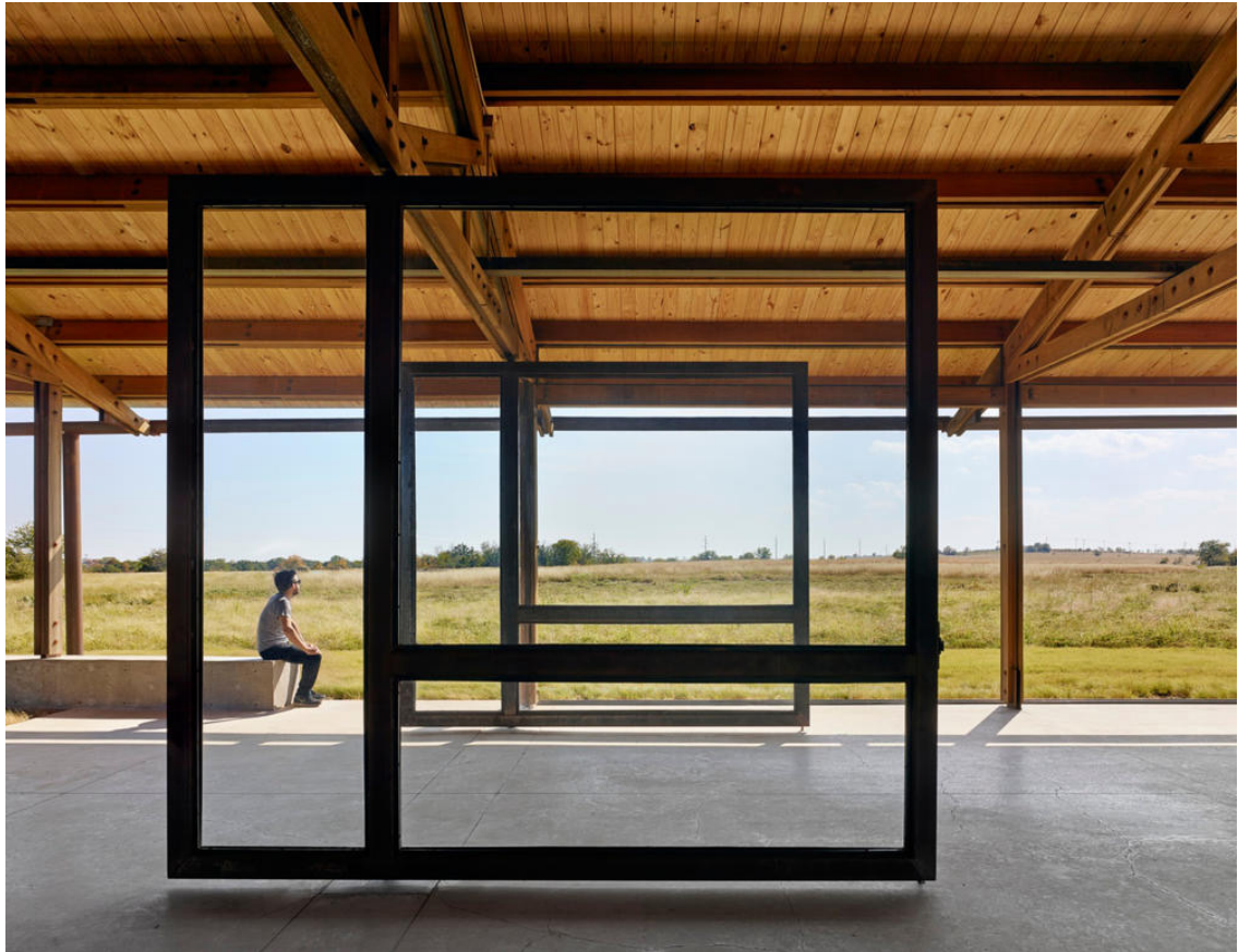
Figure 3: Non-load bearing partitions can be adapted without threatening the structural integrity of the building. 2016 COTE Top Ten Recipient Dixon Water Foundation Josey Pavilion by Lake|Flato Architects. Photo Credit: Casey Dunn
